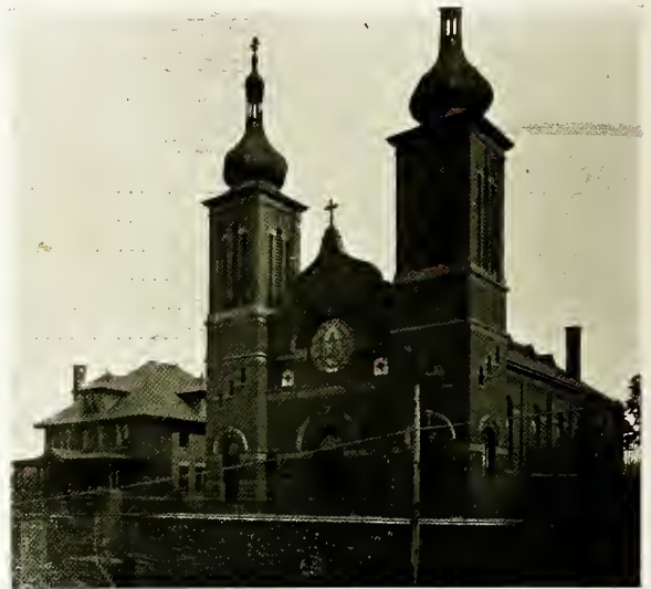
St. Mary's Greek (R. C.) Church North Main Street
